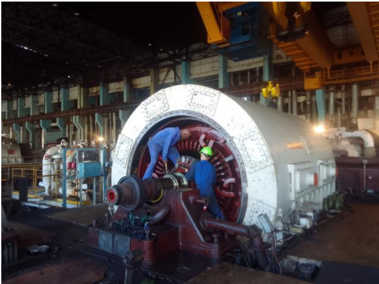
Work on a turbine at a power station (Source: Granma )
