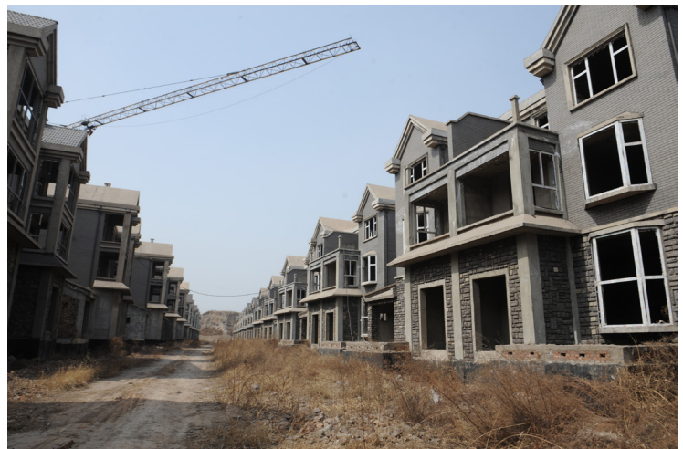
Nearly 100 villas built in 2008 lie abandoned in Taiyuan, Shanxi Province.
